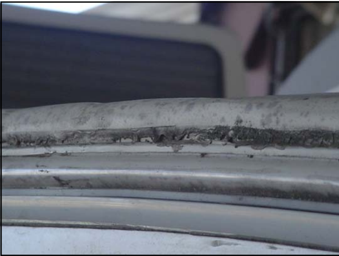
These images illustrate poorly maintained sealants.
